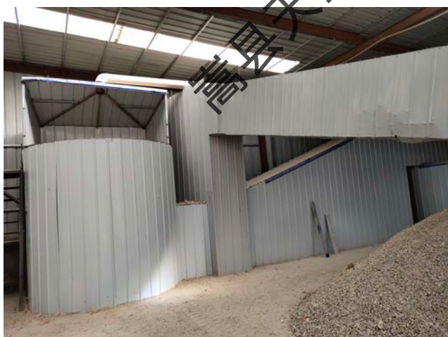
破碎机进料处设置集气罩
